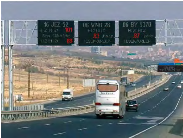
RADOR 201, Ankara - Polatlı - Sivrihisar Road, VMS with Radar and Average Speed / 2011 RADOR 201, Ankara - Polatlı - Sivrihisar Yolu Radarlı ve Ortalama Hız alan VMS
