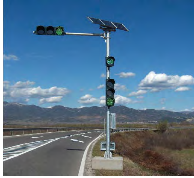
Wireless and Solar Powered Signalization System, REPUBLIC OF MACEDONIA / 2007 Kablosuz ve Güneş Enerjili Sinyalizasyon Sistemi, MAKEDONYA
