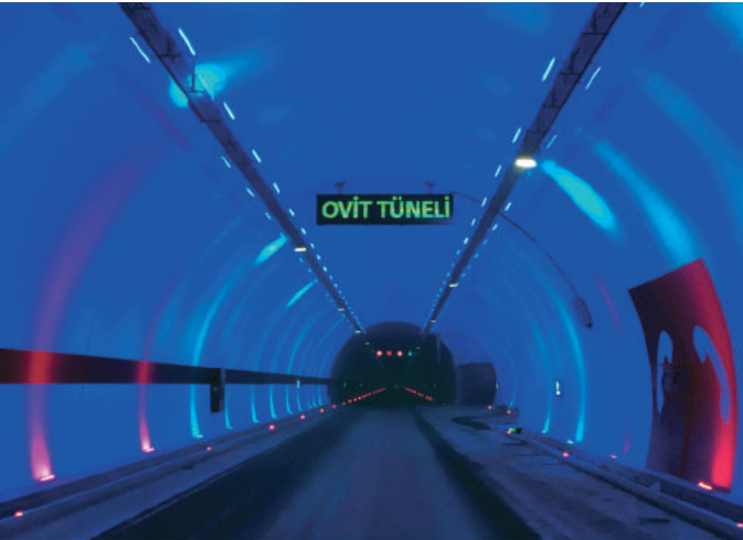
OVIT Tunnel ITS, RİZE / 2017 OVIT Tüneli AUS Projesi, RİZE
