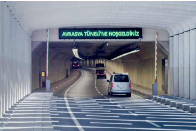
İstanbul Eurasia Tunnel, VMS / 2016 İstanbul Avrasya Tuneli, VMS
